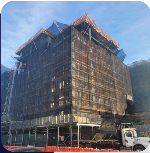
953 Dean Street SCOPE: Sidewalk Shed, Pipe Scaffolding, Hoists, Horizontal Netting, Roof Protection. New Construction by Twin Group Associates.
