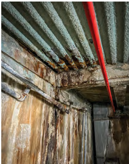
Beam Encasement Spalls
