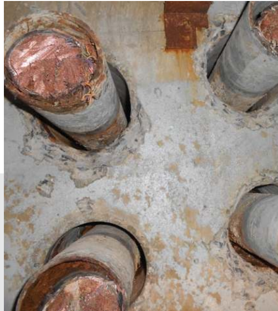
CONDUIT SLEEVE TO CABLE(S) PENETRATION (ANNULAR INJECTION)
