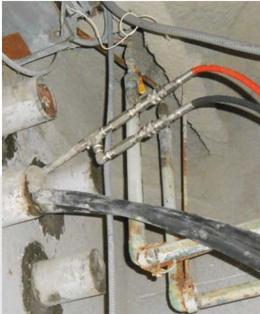
CONDUIT SLEEVE TO CABLE(S) PENETRATION (ANNULAR INJECTION)
